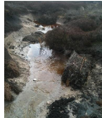
Figure 5: Broken bale dam 8 years after installation
